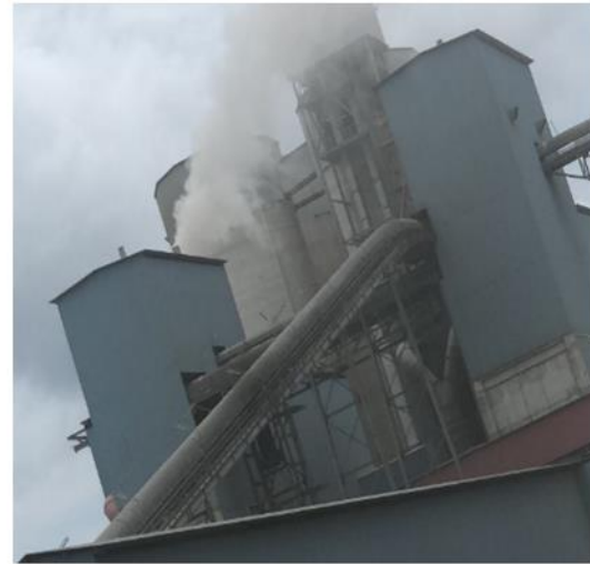
Figure 10: High cement dust emissions
