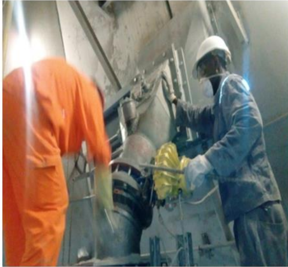
Figure 9: Cement silo (caked cement) cleaning
