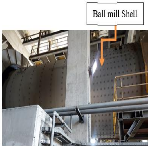
Figure 2: Installed Ball Mill Shell
