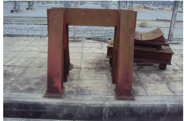
Figure 13: Pulling jack stand with saddle carriage.
