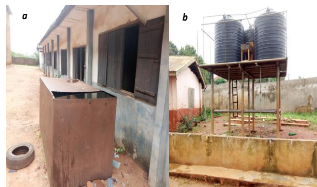
Figure 2: (a) Rain as water sources in a government school; (b) Overhead tank supply at a mission school
